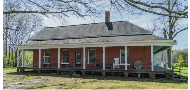
Prater house, low pitch roof with added porch roof.
